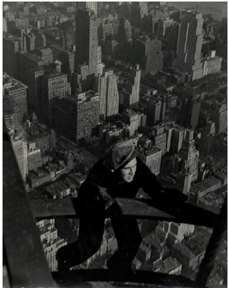
F.199. Lewis W. Hine: Worker Hanging on to Two Steel Beams (1931). / George Eastman House, Rochester, NY
